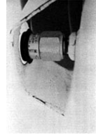
The safety valve is designed to relieve excess pressure from the vapor space of the tank at a predetermined start-to-discharge setting.
